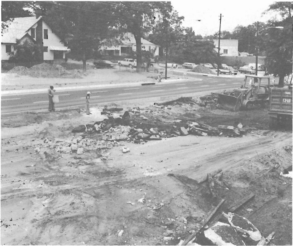
Figure 6. Monitoring grading of an abandoned street surface. Note the streetcar tracks in the foreground.
