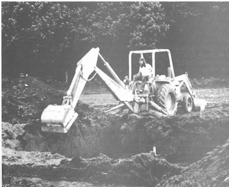
Fig. 2. Backhoe removing overburden from Early Archaic horizons.
